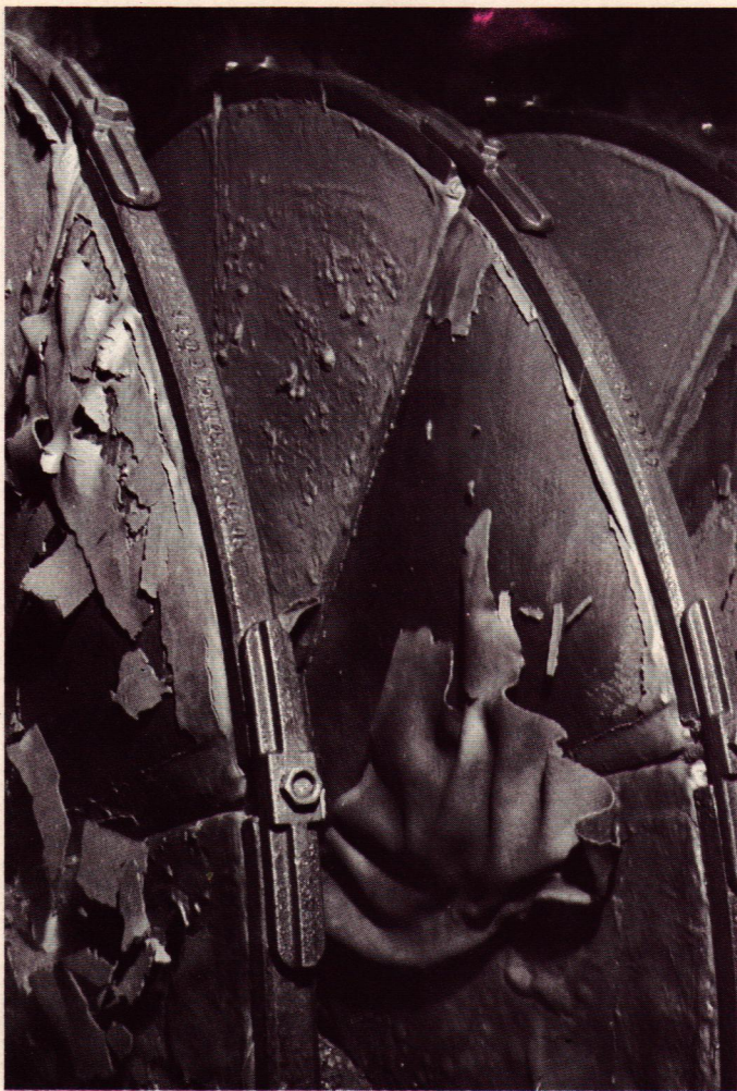
Half submerged in the slurry, these slowly turning screen-faced disc filters suck the water from the slurry and blow the semi-dry "cake" onto a conveyor.
