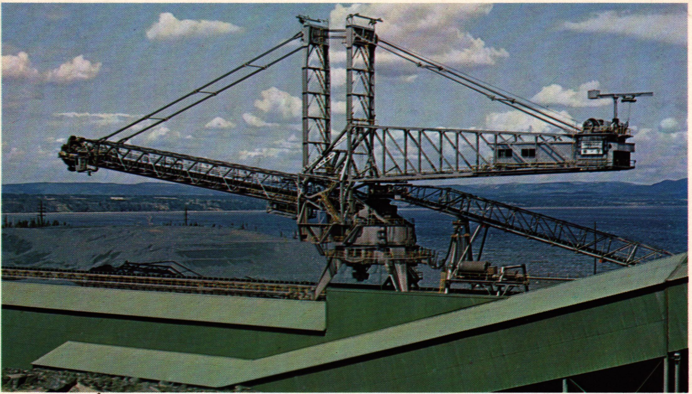
This monstrous steel machine is the stacker-reclaimer.
