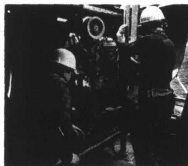
Drill shack atop a barge at Gull Island.
