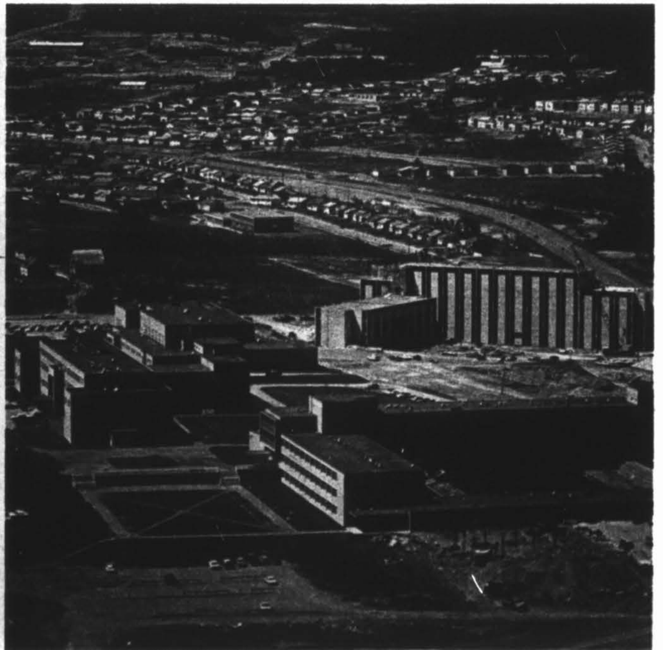
Partial view of the campus of Memorial University, St. John's.
