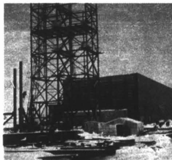
Steelwork for 26-story digester section.
