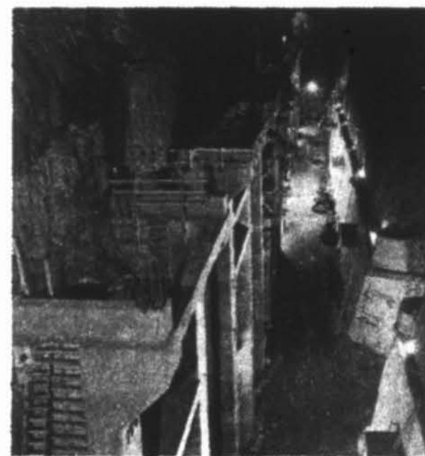
Churchill Falls underground surge chamber.
