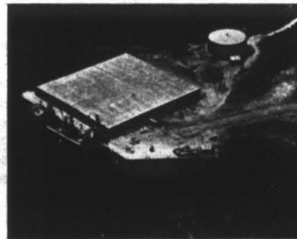
26,000 ton storage warehouse (480 foot long pier) capable of docking vessels up to 13,000 tons.
