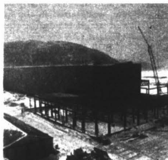
The mill building, 1/5 of a mile long.
