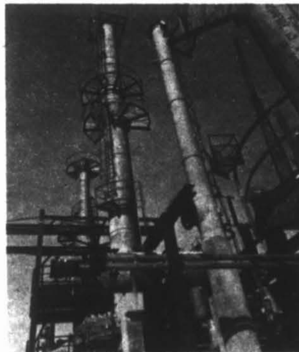
Golden Eagle refineries incorporate the latest technological advances in environmental protection.
