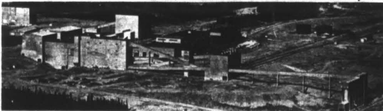
The Wabush Mines complex, which came into production in 1965, now has an annual capacity of six million tons of iron ore pellets.
