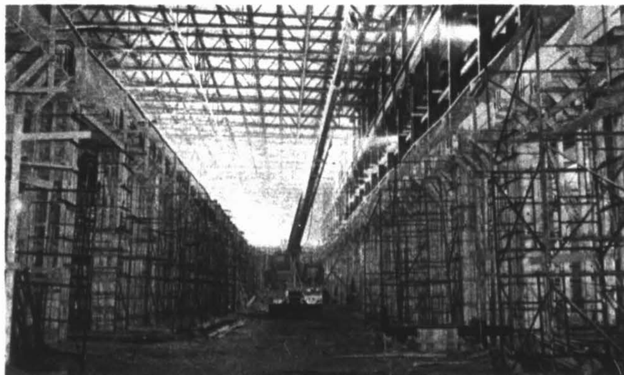
Interior of mill building where linerboard machine is being installed.
