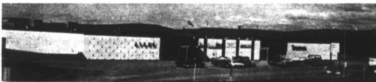
The modern Wabush shopping center features a department store, supermarket, pharmacy, electrical appliance and furniture store, post office and other convenient business places.
